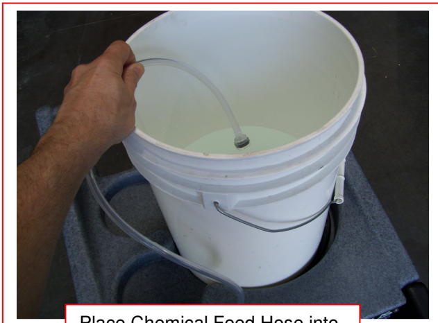
Place Chemical Feed Hose into Rinse Solution
